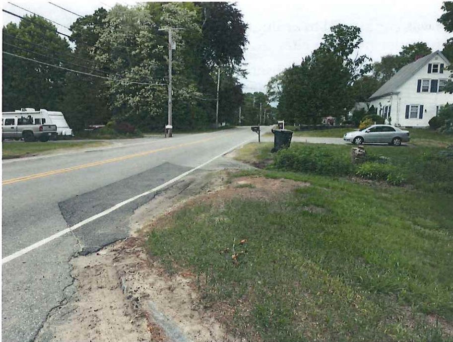
Northern curb cut looking north
