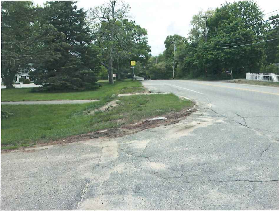
Northern curb cut looking south
